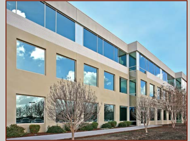
Building C reate 10911 White Rock Road
