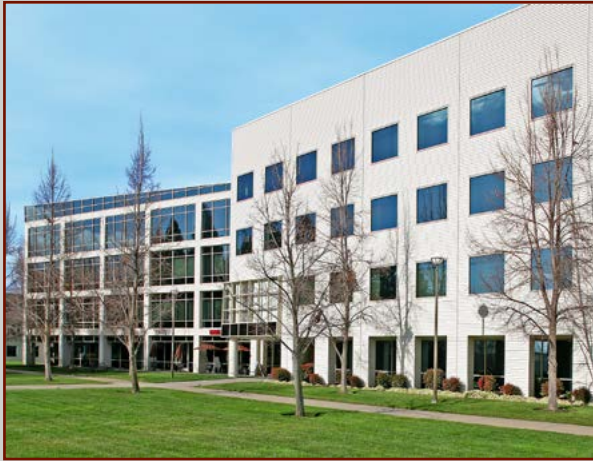
Building A spire 10860 Gold Center Drive
