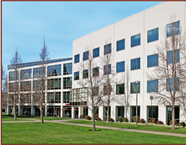
Building A spire 10860 Gold Center Drive
