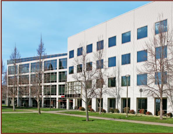
Building A spire 10860 Gold Center Drive
